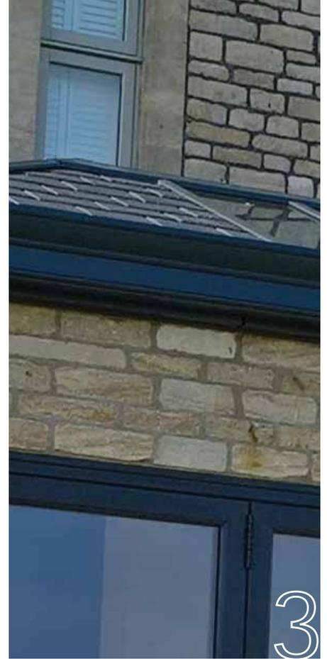
1. Insulated internal pelmet. 2. Central lighting panel. 3. Ultrarof lightweight tiled roof and curved cornice. 4. PVCu roof vent. 5. Super-insulated column with fluted infill panel and two tier flat cornice. 6. Super-insulated column with flat infill panel and three tier flat cornice.
